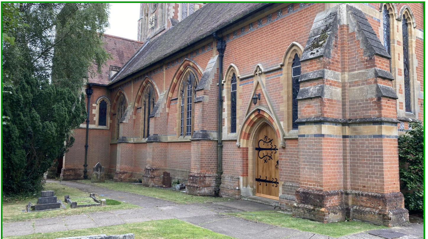
The North Wall with refurbished north door.
