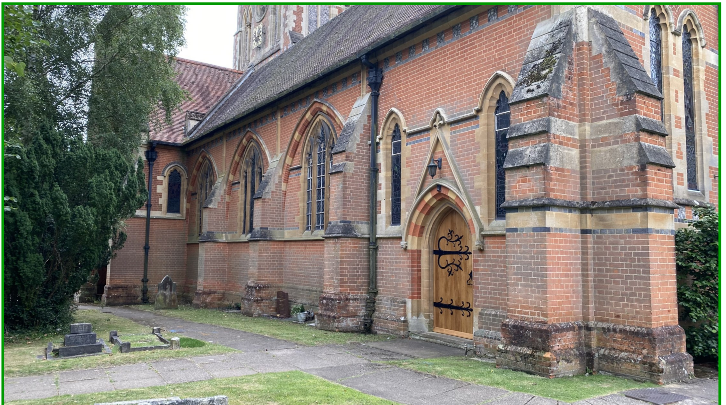
The North Wall with refurbished north door.
