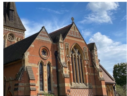
West end from NW corner
